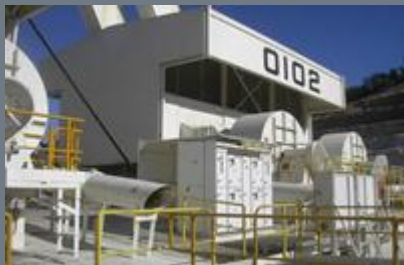
Callide - Roof Filter House
