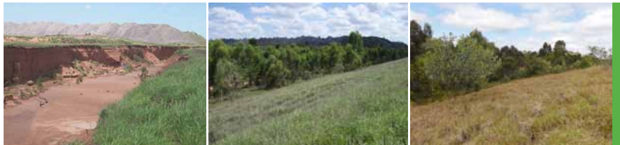
Peak Downs Mine successfully diverted Cherwell Creek. This series of photographs show how well the diversion has been maintained from initial work in 1999, 2007 and 2011. Photos courtesy of Rohan Lucas and Ross Hardie.
