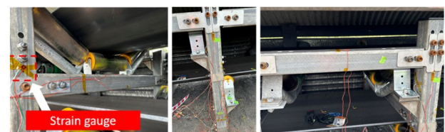
Figure 2: Strain gauges to monitor critical locations of the GFRP frames.
