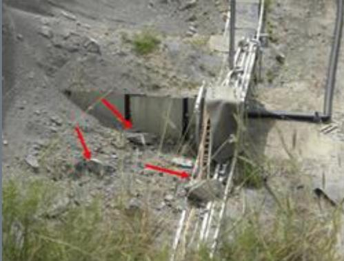
Consequences of rockfall events observed around abandoned portal entries at the base of the highwall at the Beltana mine (Glencore). Red arrows indicate larger blocks identified nearby the portals.
