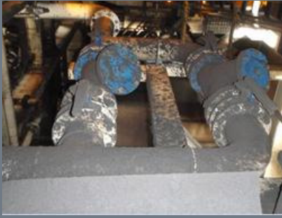
Dual back-flush strainers
